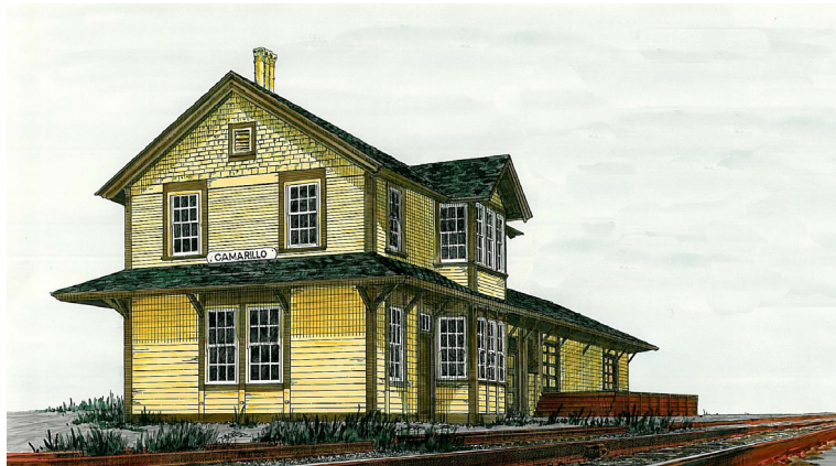
Elevated loading area, large sliding doors, one and two story elements, and deep set eaves.
