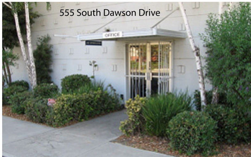
The building finish floor is very close to top of street curb elevation.
