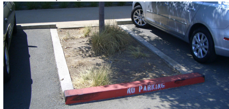
Water runs from sidewalk and parking surface into planter area.
