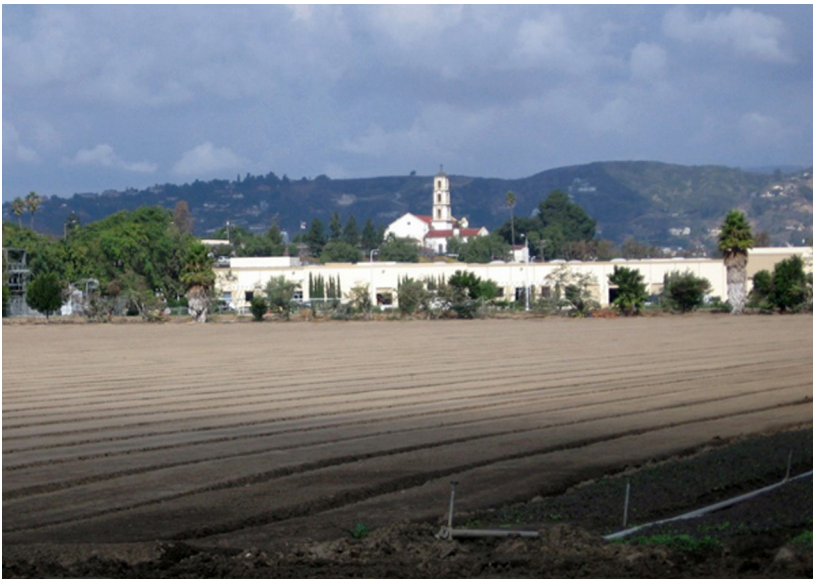
EJM property looking north to a portion of the Imation property.
