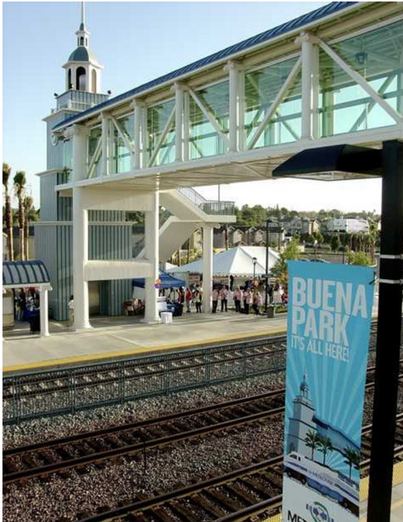
This grade separated crossing is serviced by elevator and an enclosed crossing span. The capital and maintenance cost for this type of crossing are considerable when compared to the existing facility in Camarillo.
