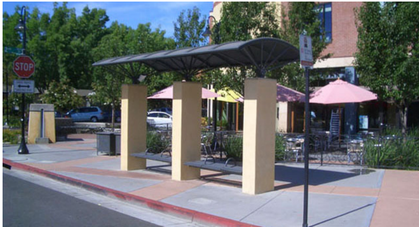
Example of a covered bus shelter.
