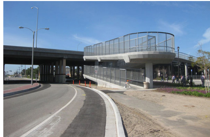
Existing pedestrian/bicycle crossing is minimally used because of the required length of travel, change in grade, and the unpleasant environment (weather, noise, and air quality) due to its proximity to Highway 101.
