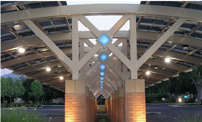
Carport with solar panels.
