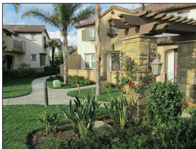
RPD 174-2 Villas at the Park Apartments
